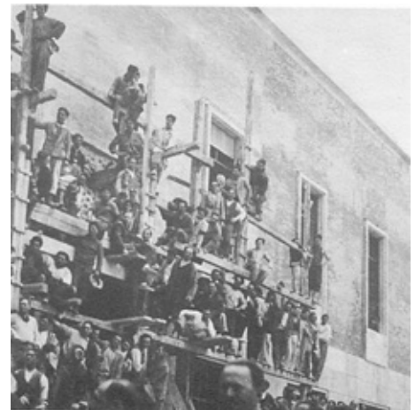
B. Workers on scaffolds, listening to Mussolini's speech during his visit at the construction site for Sabaudia. 18 Dec. 1933.
