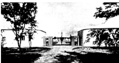
C. (below): Entrance gate to the cemetery.
