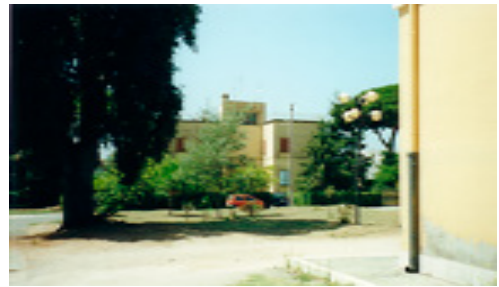
B. View of the villa from the Agricultural Concern's courtyard.
