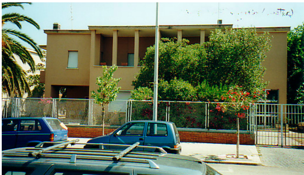
C. Photo of the façade, present state.
