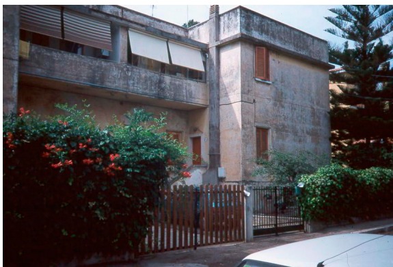
B. Photo of the façade facing the street.
