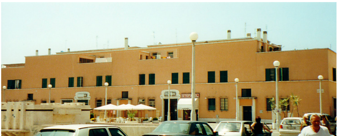
A. Photo of façade facing the square.
