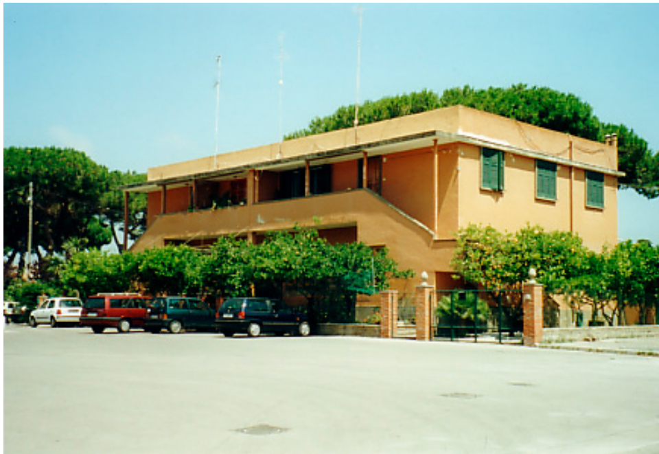
A. The building, seen from the ONC courtyard.
