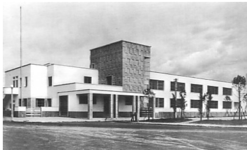
C. Photo of façade.
